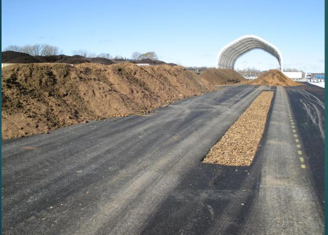
Loaded batch at left and open zone to right. Windrows typically 18 ft. wide and 8 ft. high. Chips are checked between batch loads for compaction and packing of wet material. Full replacement every 3-5 years.
