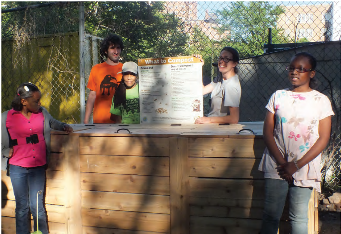
Volunteers pose behind a newly constructed three-bin compost system at Chenchita Community Garden in Manhattan.
